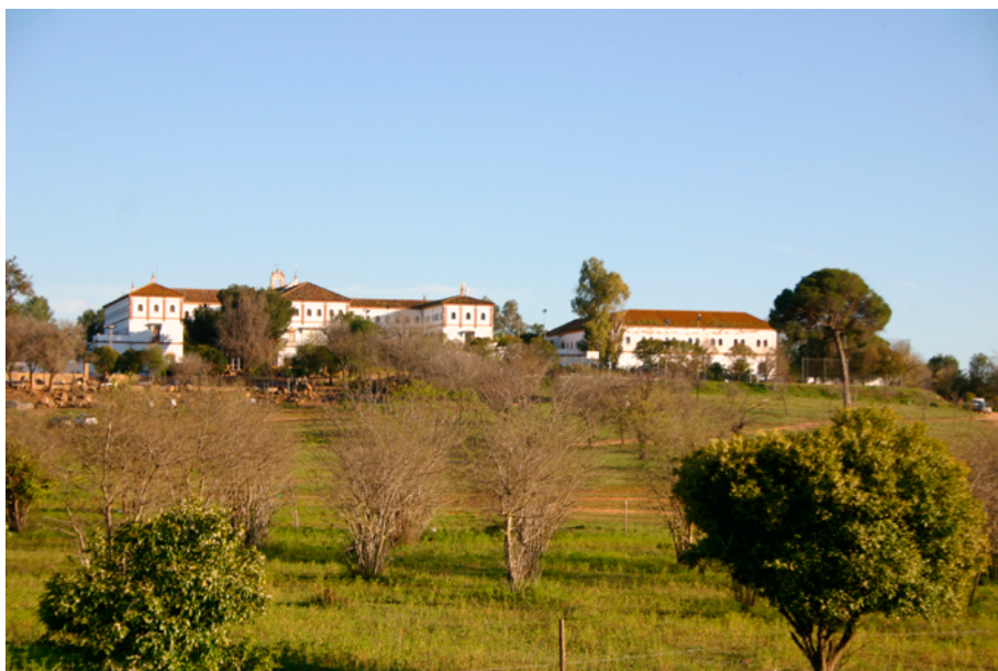
FIG. 3. Reformatory of Alcalá de Guadaíra. The left module formed by three pavilions is work of Juan Talavera Heredia; the right, of Aurelio Gómez Millán. (Photo author).
